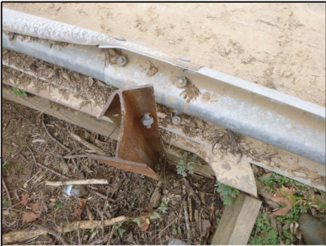
DAMAGED BRIDGE RAIL POST REPLACE WITH NEW POST (SEE RAIL POST DETAILS BELOW)
