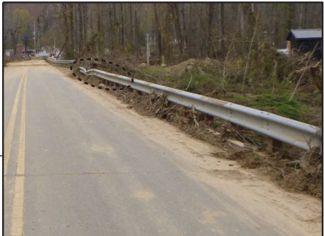
12-FOOT LONG SECTION OF BRIDGE/ GUARD RAIL DAMAGED TO BE REPLACED
