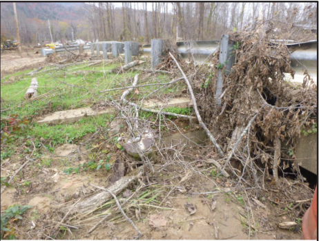
3"x10"-10' LONG TOP TIMBER WING BOARD DETACHED REINSTALL OR REPLACE
